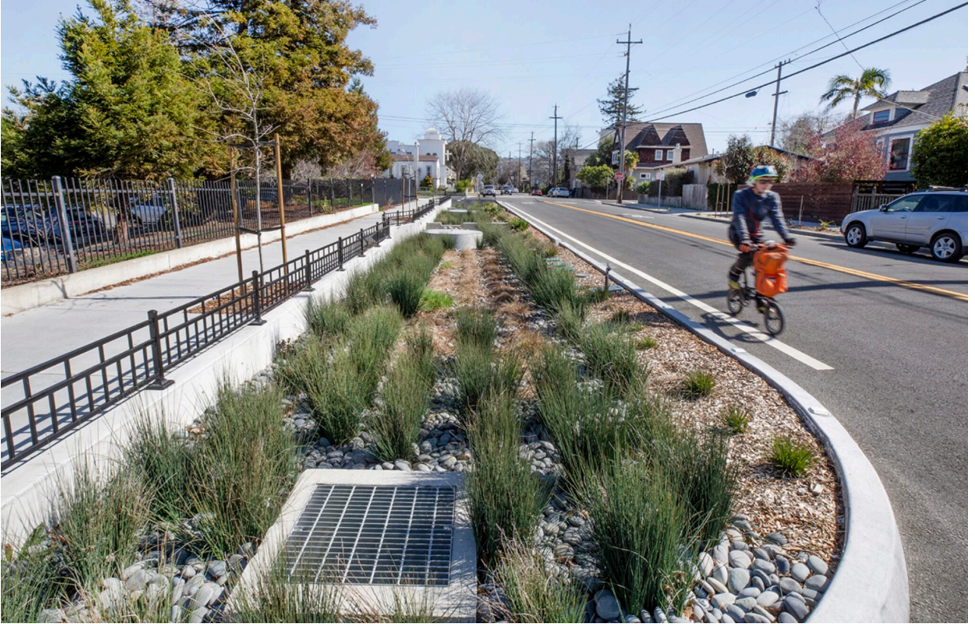
Berkeley Springs Downtown Green Infrastructure Retrofit
